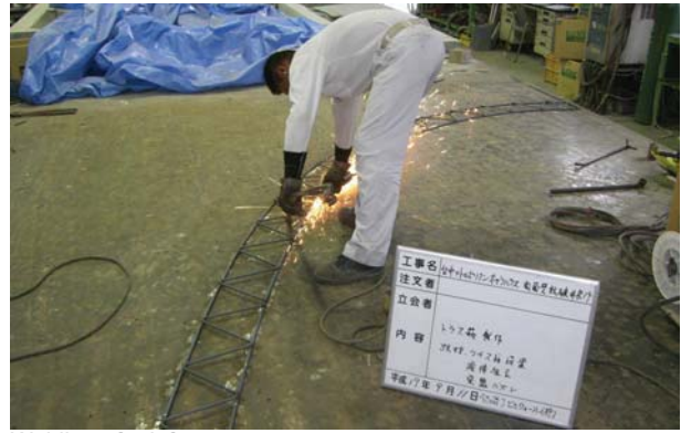
Welding of reinforcement truss
