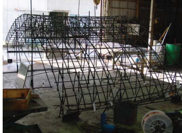
Pre assembled Truss wall
