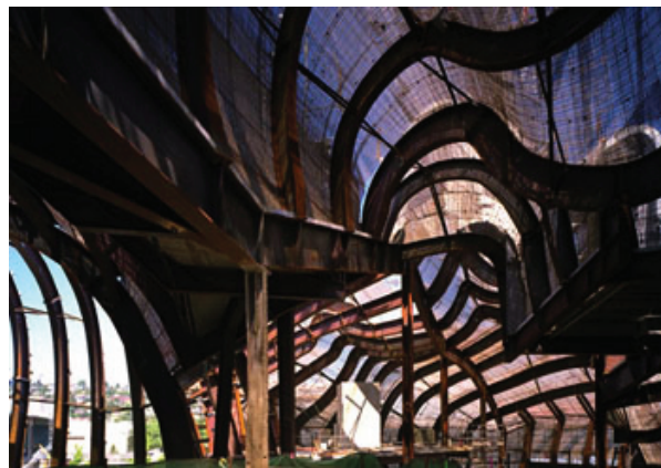
Figure 4: Structural frames in Frank Gehry's Experience Music Project in Seattle, produced by contouring (Kolarevic 2001).
